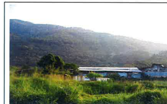
Photo No. C6-I6 Temporary Structure for poultry and Open Storage at upstream of Ma On Kong Channel
