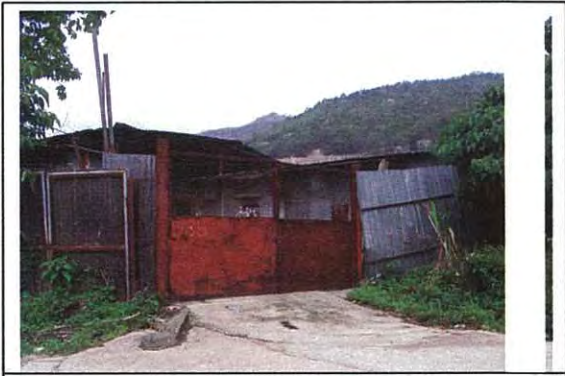
Photo No. B12—LCA 6 Industrial Landscape Character Area
