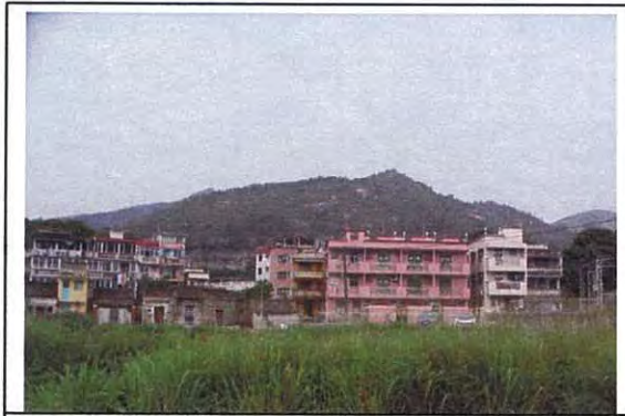
Photo No. C10—R3
