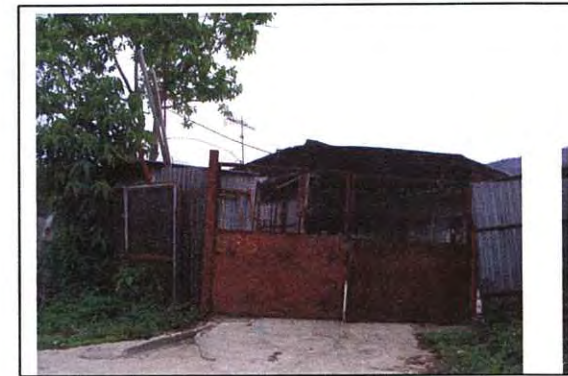
Photo No. B12—LCA 6 Industrial Landscape Character Area
