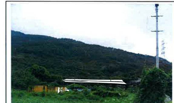
Photo No. C6—I6 Temporary Structure for poultry and Open Storage at upstream of Ma On Kong Channel
