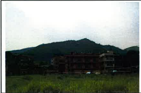
Photo No. C10—R3
