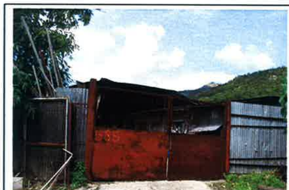
Photo No. C5-I5 Open Storage at the end of village access road
