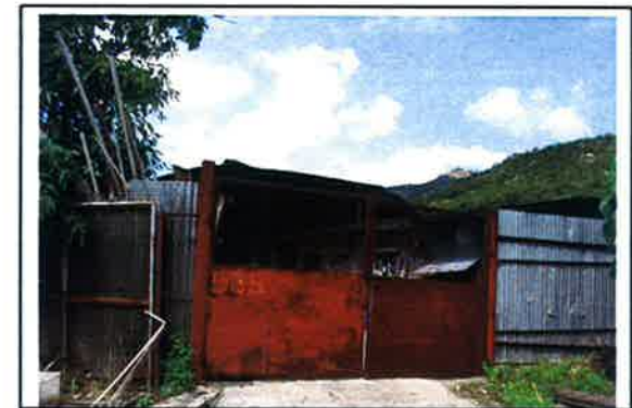
Photo No. B12—LCA 6 Industrial Landscape Character Area
