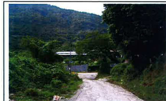
Photo No. C6—I6 Temporary Structure for poultry and Open Storage at upstream of Ma On Kong Channel
