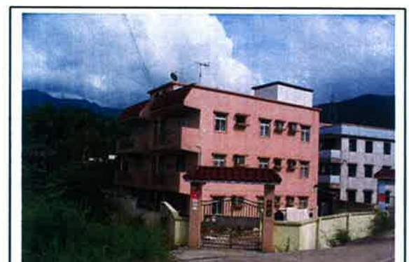
Photo No. C9 – R2 North of Ma On Kong
