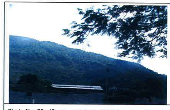
Photo No. C6—16 Temporary Structure for poultry and Open Storage at upstream of Ma On Kong Channel
