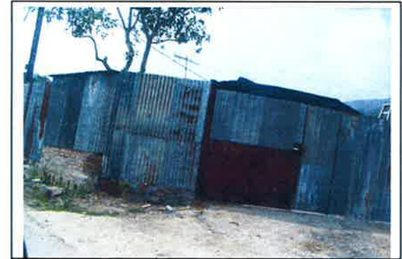
Photo No. B12—LCA 6 Industrial Landscape Character Area
