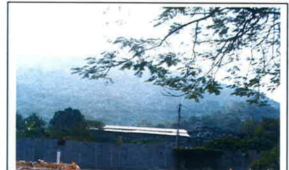
Photo No. C6—I6 Temporary Structure for poultry and Open Storage at upstream of Ma On Kong Channel
