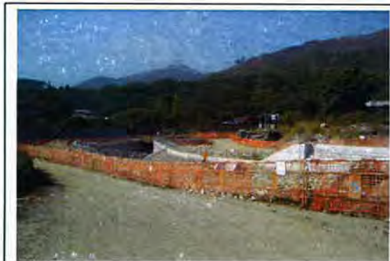
Photo No. B8 – LCA4 Fish Pond Landscape Area
