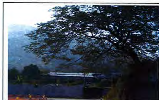
Photo No. C6—I6 Temporary Structure for poultry and Open Storage at upstream of Ma On Kong Channel
