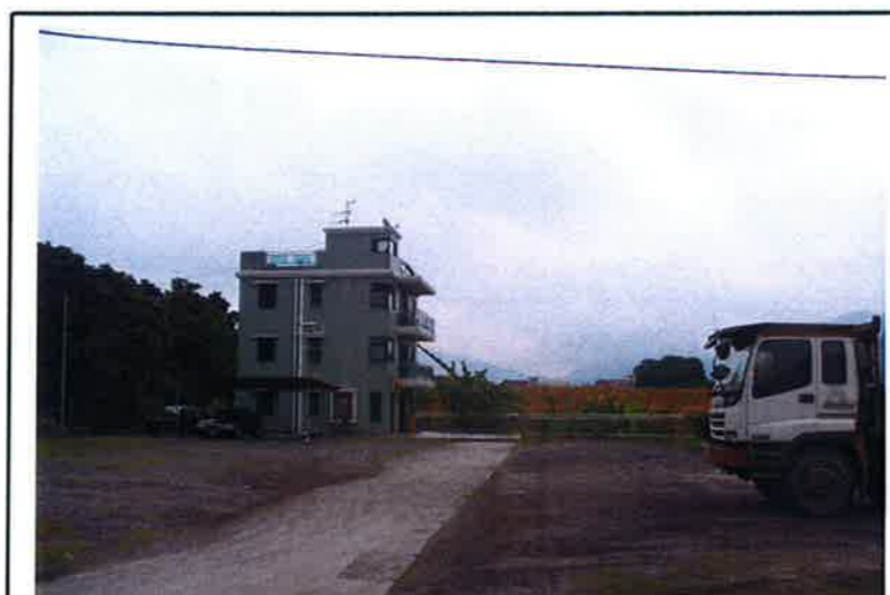
Photo No. C2—I2 Plant Nursery at the east of Ma On Kong Channel
