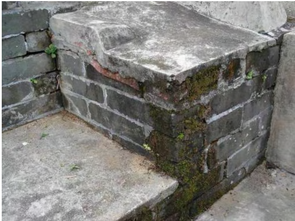
Figure 3.2f Condition of cement mortar of grave bricks at the right hand side of the headstone. Cement mortar and bricks are covered with overgrown vegetation (photo taken on 9 January 2010).
