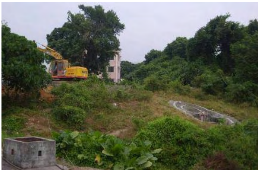
Figure 3.2b A platform was being constructed adjacent to the grave with an excavator moving around it (photo taken on 4 Nov 2009).
