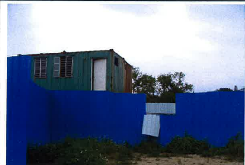
Photo No. C4—I4 Temporary Structure for poultry east to Ho Pui
