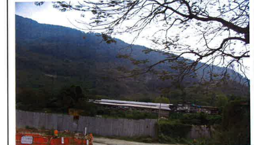
Photo No. C6—I6 Temporary Structure for poultry and Open Storage at upstream of Ma On Kong Channel
