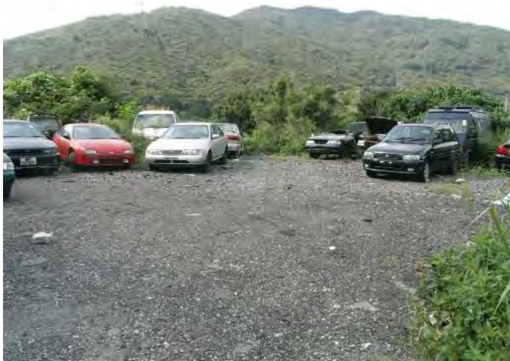
Figure 3.4 General view of the platform used as a car park (photo taken on 25 June 2011)
