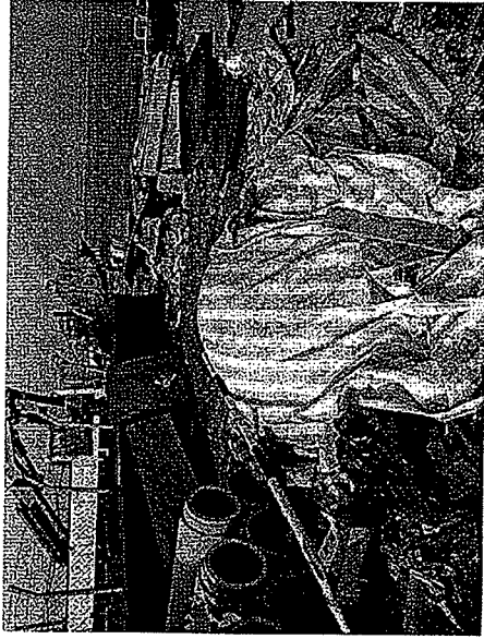
Photo_120111_002 (Some construction waste materials noted in Portion J were collected)
