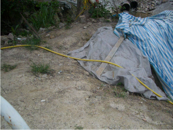
General refuse is cleaned from TKL-07.
