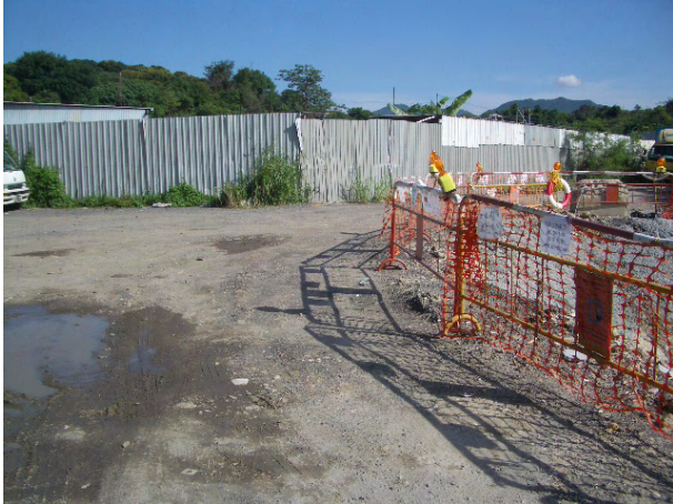
Stagnant water at TKL-07 was cleared.
