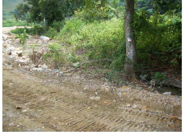
Stagnant water is cleared at TKL07.
