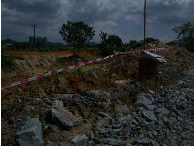
C&D removed and channel diverted at TKL02.
