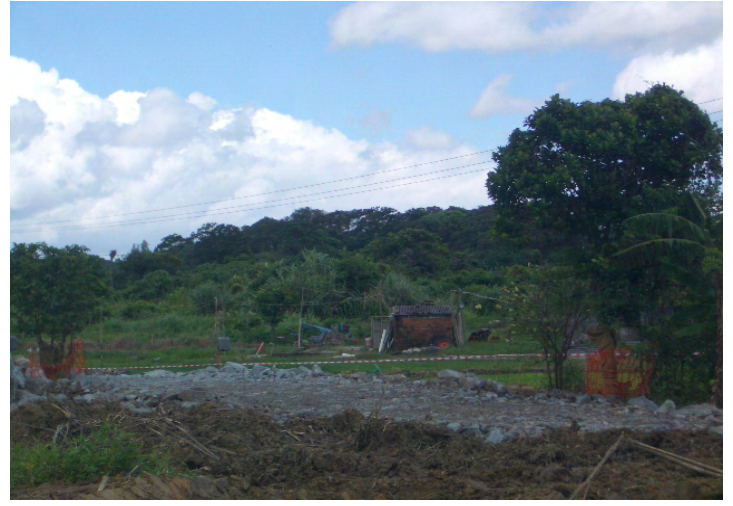
Preserved trees are properly fenced at TKL02.
