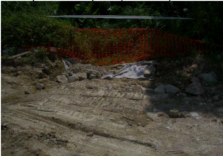
Desilting facilities implemented at TKL02.
