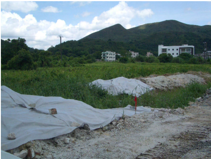
Exposed slope was properly covered at MUP01/02.
