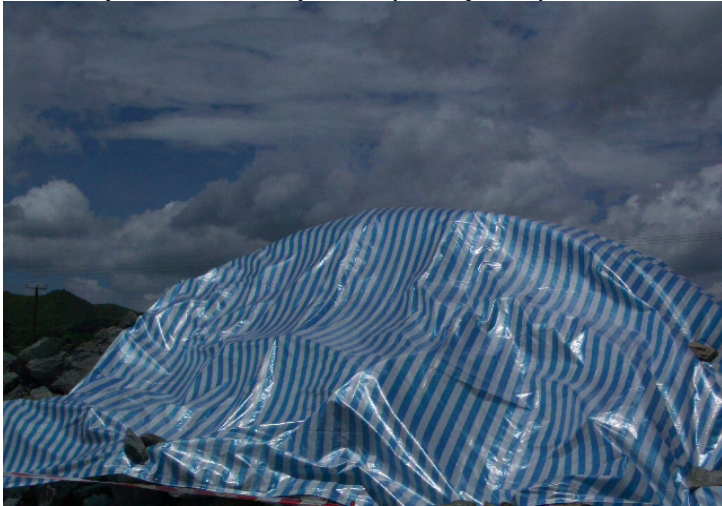
Stockpile was covered with tarpaulin at TKL02.
