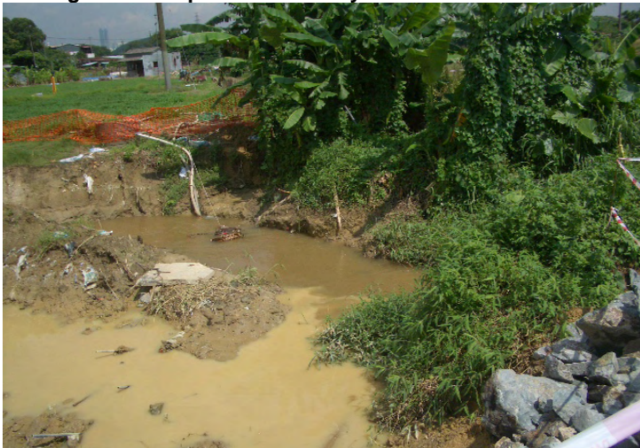
1. Muddy water to be treated before discharge at TKL02 . The contractor is advised to remove the muddy water, and implement certain mitigation measures.
