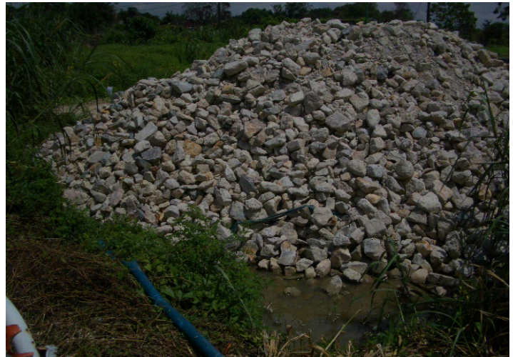
Muddy water was desilted prior discharge at TKL07.
