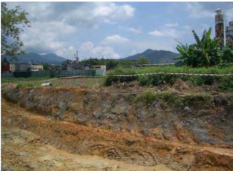
Cut-off slopes was protected by cement soil
