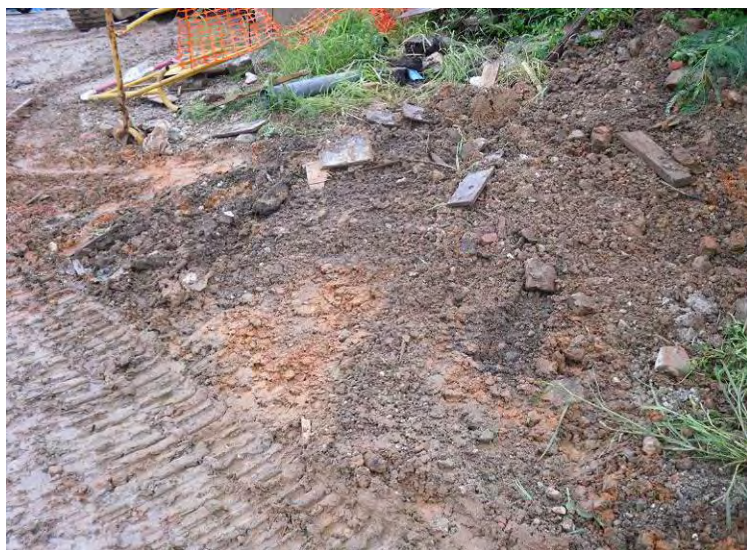
C&D wastes have been removed at TKL07.
