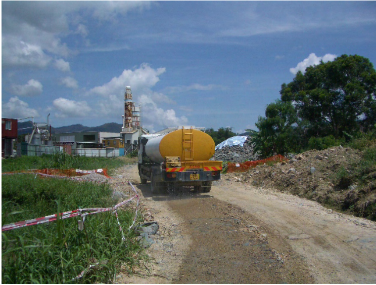
Water spraying for the site haul road has been practiced.
