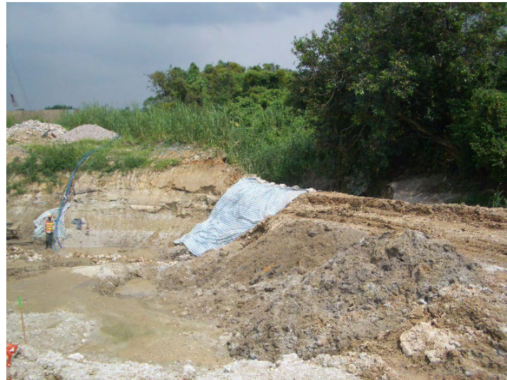
Damaged earthbund has been rectified at TKL07.
