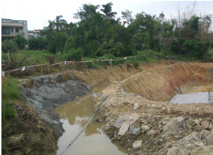
Damaged earthbund has been rectified at TKL02.
