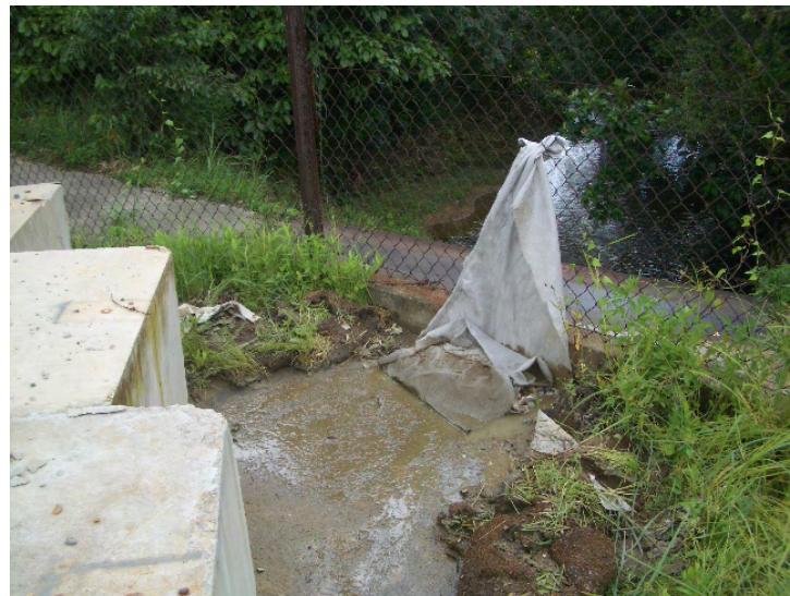
Filter has been set up at MUP01/02 to prevent surface runoff.
