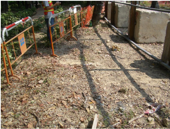
Paint containers were cleared at MUP05.
