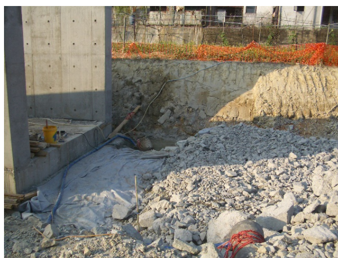
Debris was cleaned up at MUP01/02
