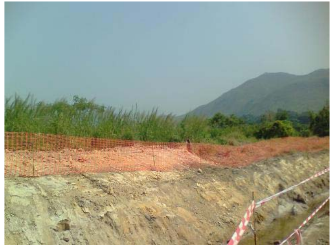
Soil stockpile was removed at TKL07.
