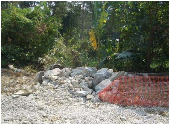
Stagnant water was cleared at MUP01/02.
