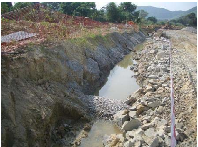
Crushed stones were paved along TKL02.
