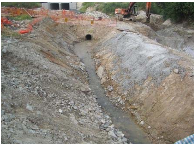
Slope was stabilized at TKL07.
