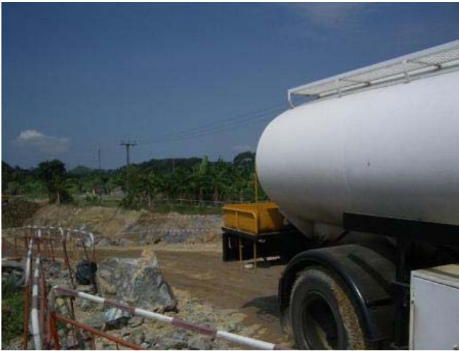
Water spraying was practiced regularly at TKL02.
