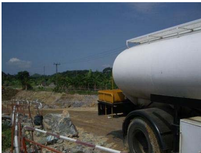
Water spraying was practiced regularly at TKL02.
