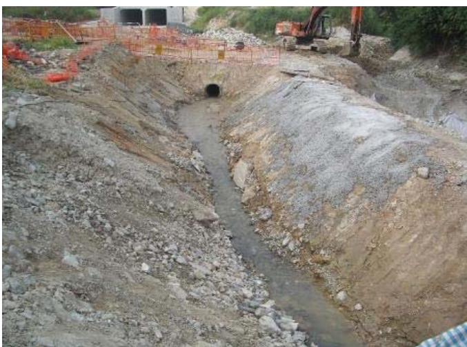
Slope was stabilized at TKL07.
