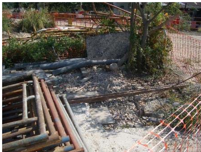
Oil containers were removed at TKL07.
