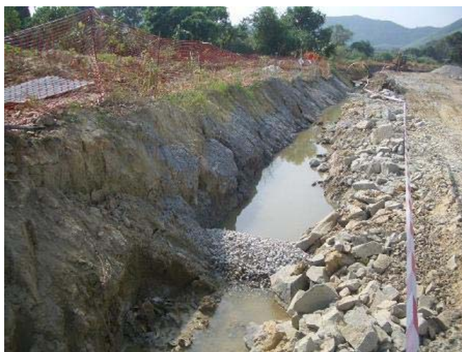
Crushed stones were paved along TKL02.
