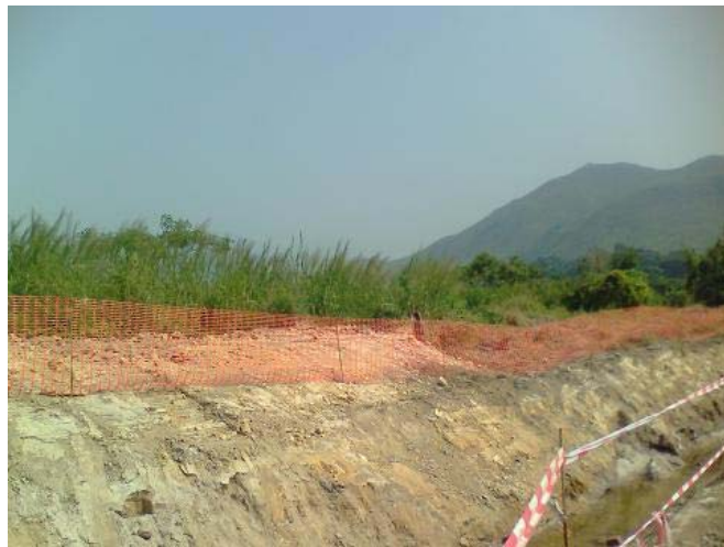
Soil stockpile was removed at TKL07.
