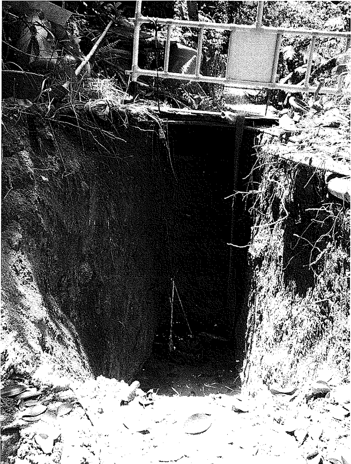
Plate 2: Deeper excavations at MH S52 – view looking west
