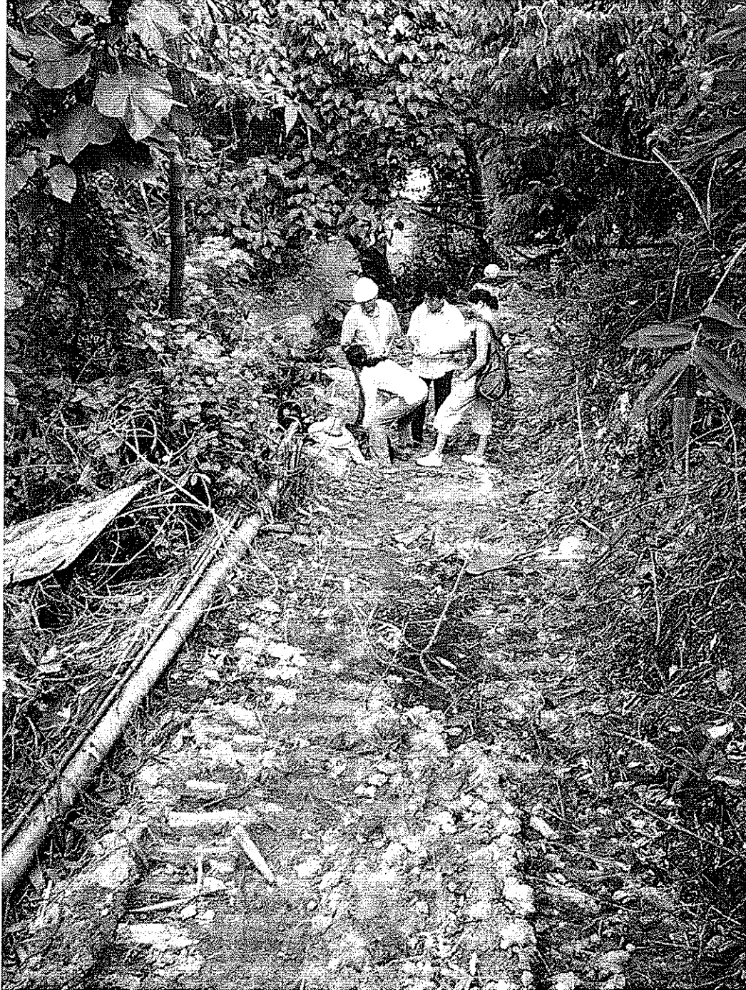
Plate 1: Pre-excitation view of the alignment between MHs S52 and S54 – looking north
