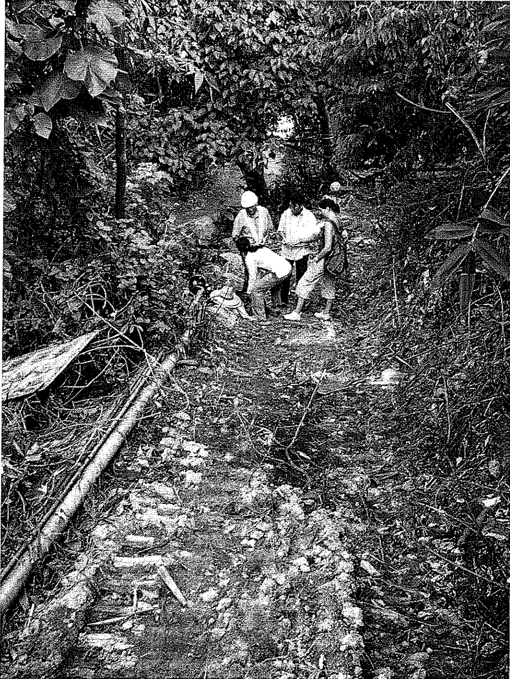
Plate 1: Pre-excavation view of the alignment between MHs S52 and S54 – looking north
