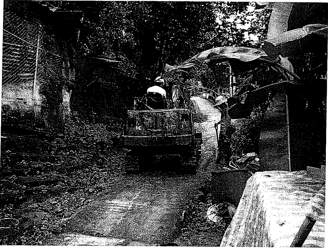
Plate 2: Pre-excitation view of alignment between MHs S51A and S50 – looking south
