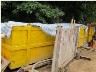
The capacity of the de-silting tanks should be improved. The Contractor was advised to provide sufficient numbers of de-silting tank for wastewater treatment in order to improve the quality of the discharge water.
