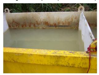
The de-silting tanks should be improved. The Contractor was advised to provide more filter sheet within the tank for wastewater treatment in order to improve the quality of the discharge water. Follow up: Rectified on
