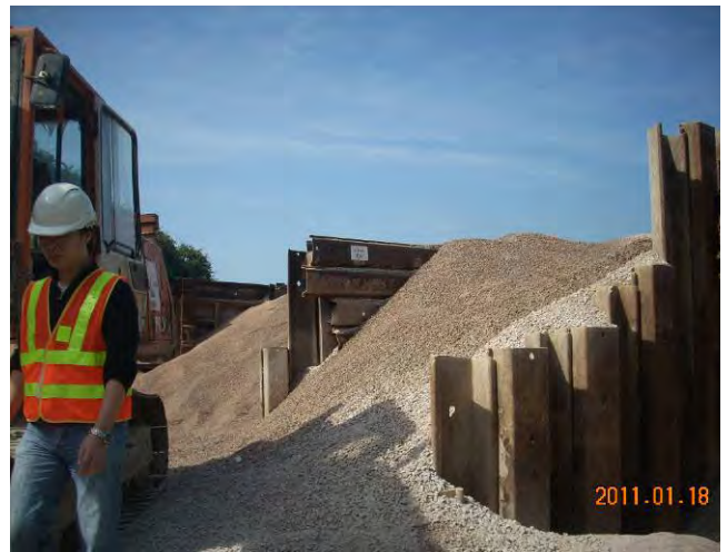
Sprinkling was applied.
