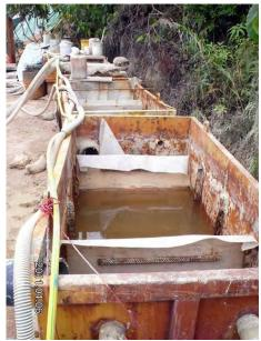
The geotextile sheets in the sedimentation tank should be properly installed to ensure the desilting function.
