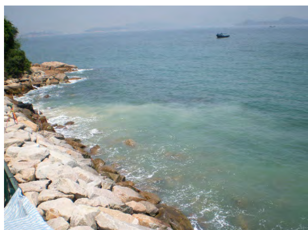
Turbid water was observed at the outfall of the site. The Contractor should carry out immediate action to avoid turbid water discharging.
