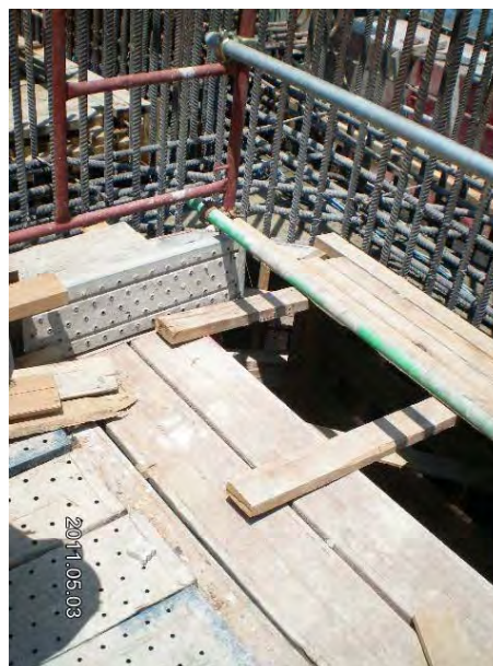
The container was taken to proper storage area. (Rectified immediately on same day)
