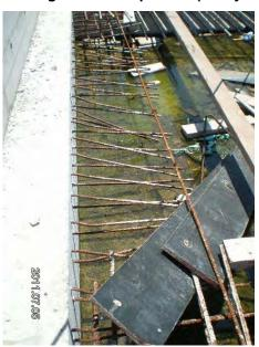
Stagnant water was accumulated on the roof of building structure. The Contractor should drain away stagnant water or apply larvidical oil to avoid mosquito breeding.
