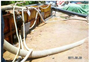
Water leakage was observed. The Contractor should repair the pipeline to avoid stagnant water accumulation.
