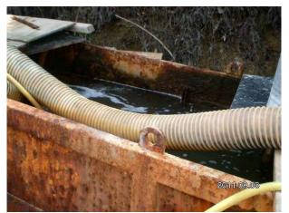
There is no geotextile sheets installed in the sedimentation tank. The contractor should install them to restore desilting functioning.
