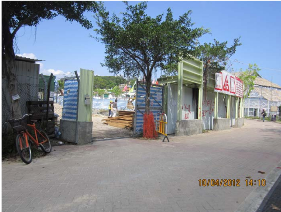
Photo B1: Dusty public road outside the site
