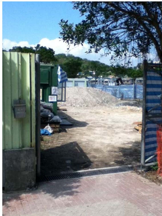
Photo B2: Stockpiles inside the site
