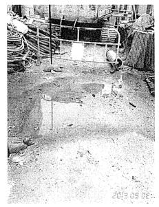
Oil leakage on the ground was observed at Yung Shue Wan pumping station, the contractor was requested to clean as soon as possible and provide proper mitigation measures to prevent further leakage.
