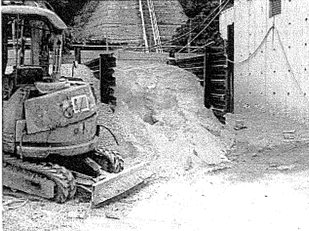
Photo 1 Stockpile of dusty materials was observed at the entrance of the pumping station, the Contractor was rounded to spray water to avoid the spread of dust.
