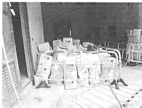
Housekeeping condition has been improved.
