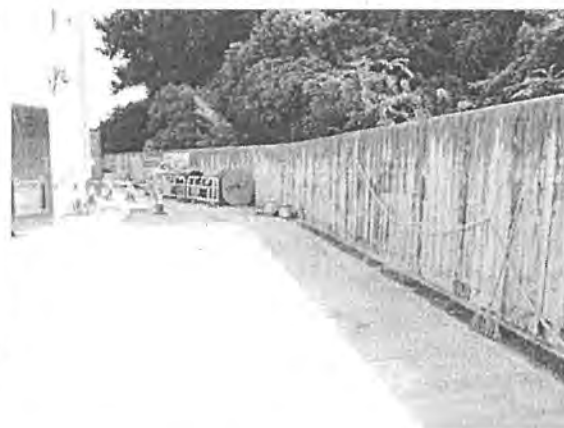
The stockpile has been backfilled.
