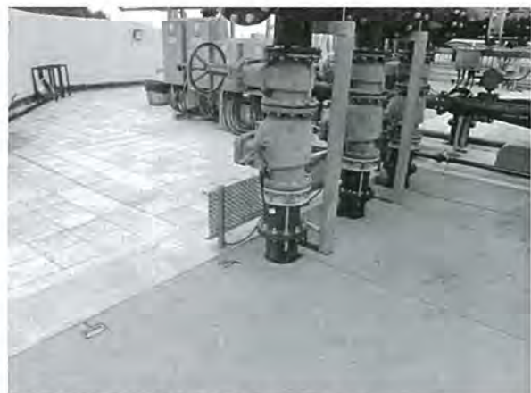
No leaking of water was observed.
