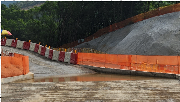
Construction of new wheel washing facility completed
