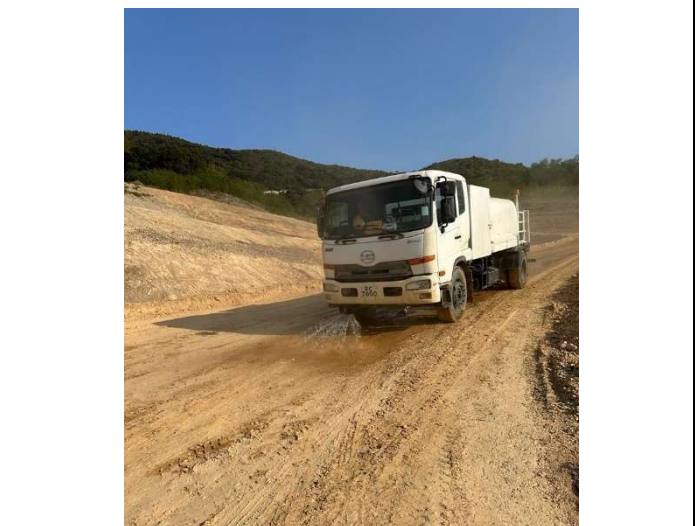
Photo 6 Water spraying by water tanker along the haul road between Portion A and the SBA
