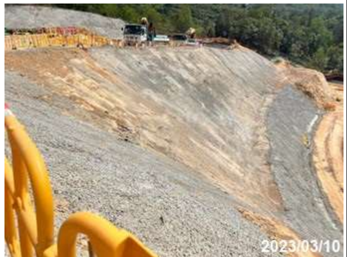
Photo 18 Application of cement slurry at Portion A
