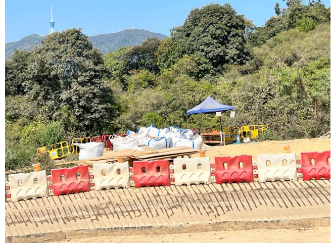
The cement bags were removed.
