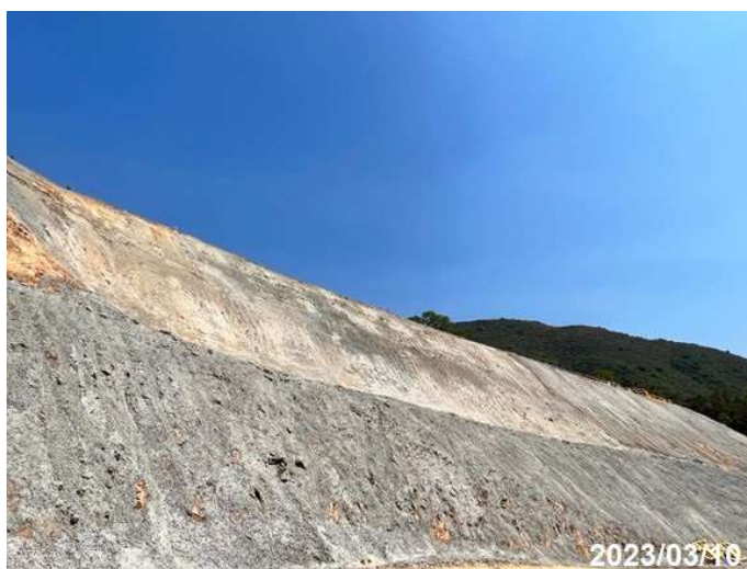
Photo 19 Application of cement slurry at Portion A
