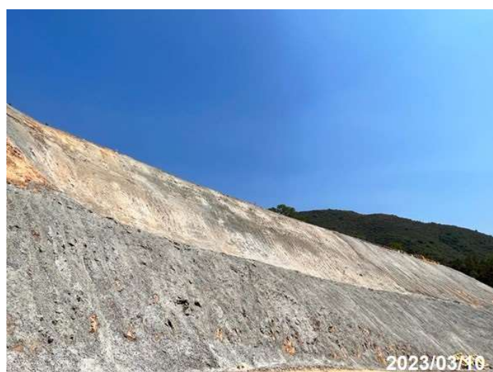
Photo 13 Application of cement slurry at Portion A
