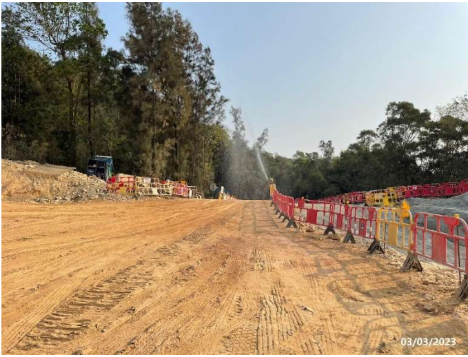
Photo 7 Water spraying by water sprinklers at Portion A
