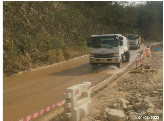
Photo 16 Water spraying by water tanker along the haul road between Portion A and the SBA
