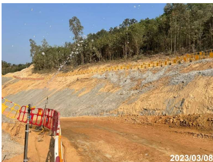
Photo 5 Water spraying by water sprinklers at Portion A
