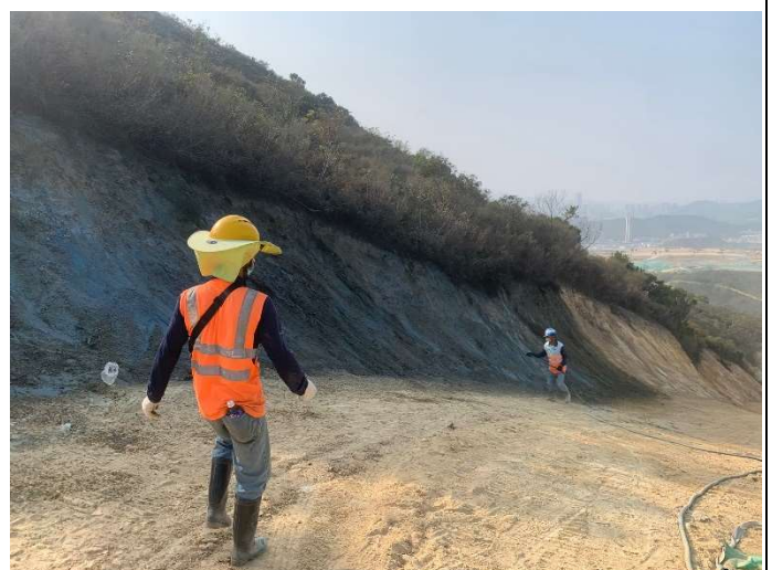
Photo 12 Hydroseeding at bare slope at Portion E3-2 (Implemented start on 26 February 2023)
