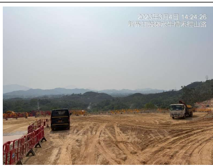
Photo 1 Site Formation at Portion A
