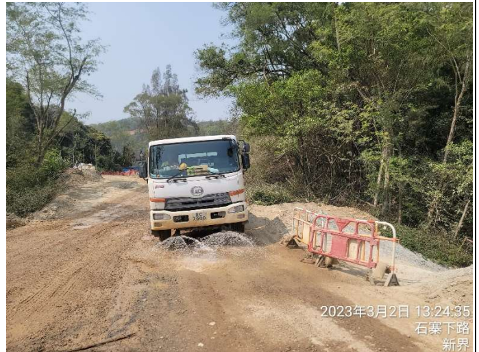
Photo 10 Water spraying by water tanker along the haul road between Portion A and the SBA
