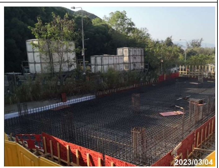
Photo 2 Permanent Building Foundation at Portion D
