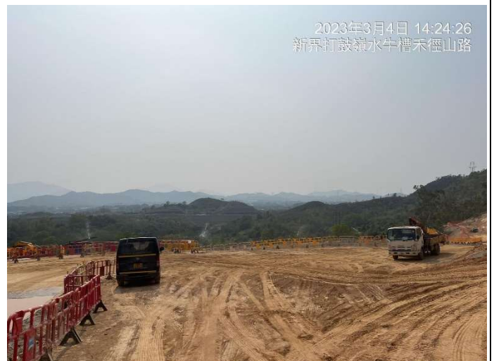
Photo 2 Site formation at Portion A
