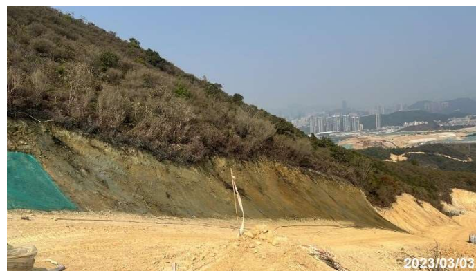
Photo 10 Hydroseeding at bare slope at Portion E3-2
