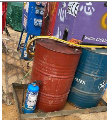
The Contractor drained off the water in the drip tray. Sand and silt in drip tray should be cleared off.
