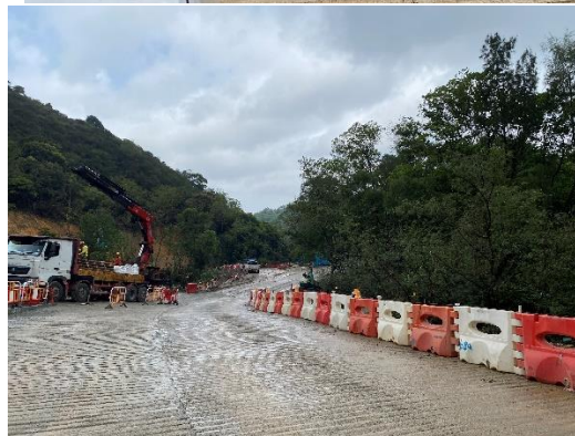
Sand and silt were removed at the entrance of SBA.
