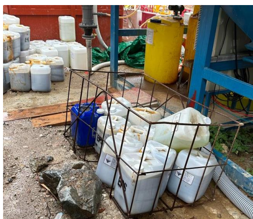
3. Chemical containers are observed in the open area and some of them are not placed inside the drip tray.
