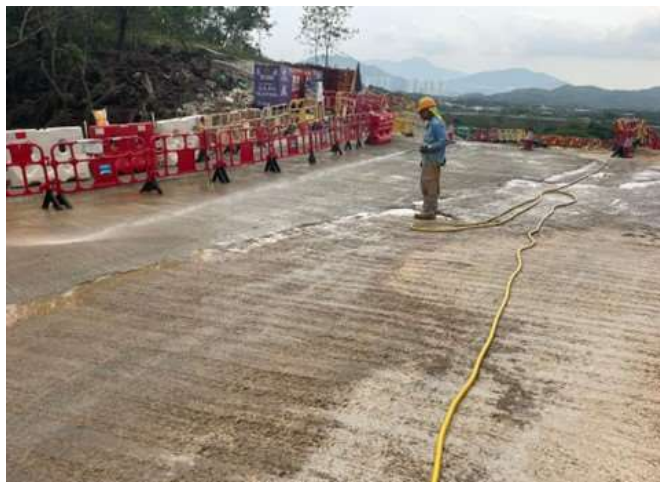
The Contractor scheduled watering at the entrance of Portion A.
