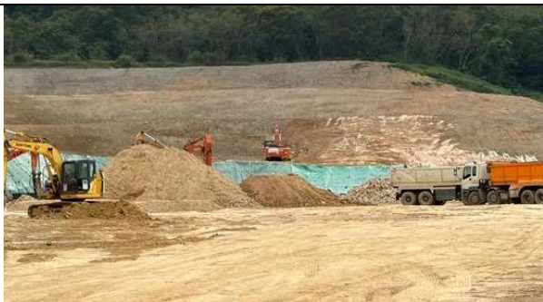
3. The Contractor was reminded to spray water on the surface of dusty material in SBA to prevent dust dispersion.
