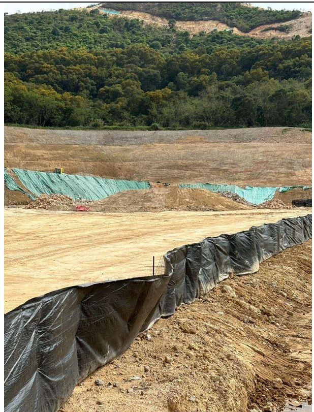
Photo 8 Portion B1 Cut-off drain with Silt fence
