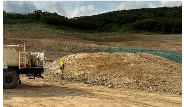
The Contractor scheduled watering for the dusty stockpile.
