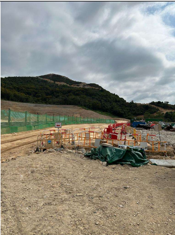
Photo 7 Portion B1 Silt fence at the soil stockpile areas
