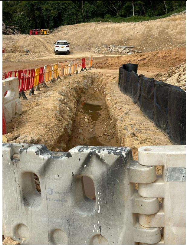
Photo 8 Portion B1 Cut-off drain with Silt fence
