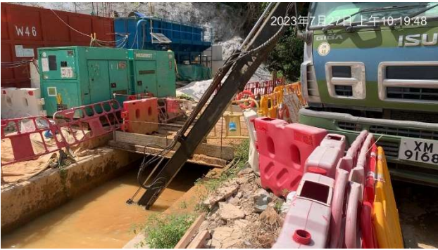
Culvert Cleaning
