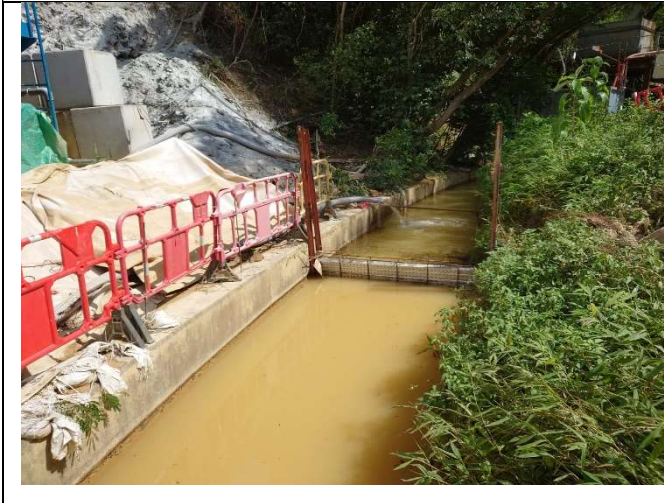
Photo 13 Channel at Portion E3-1
