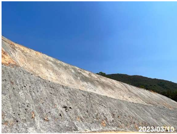
Photo 14 Application of cement slurry at Portion A
