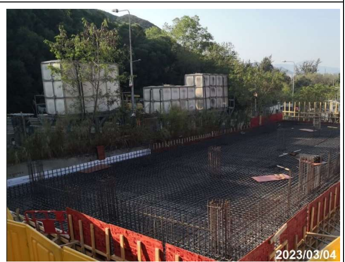
Photo 2 Permanent Building Foundation at Portion D
