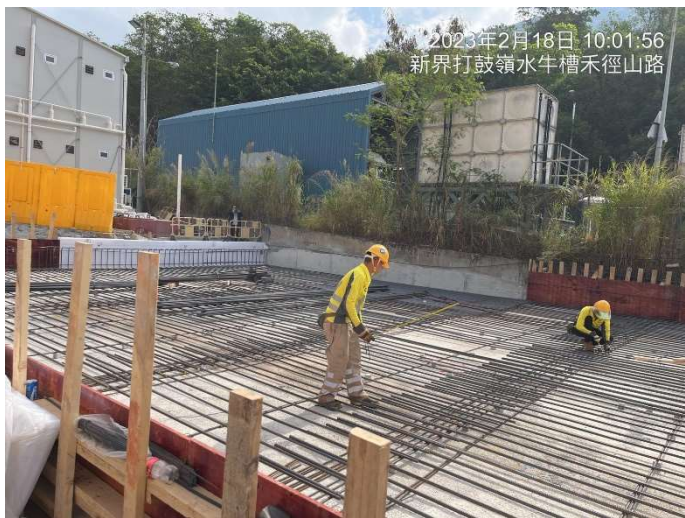
Photo 3 FSB Rebar Fixing at Portion D
