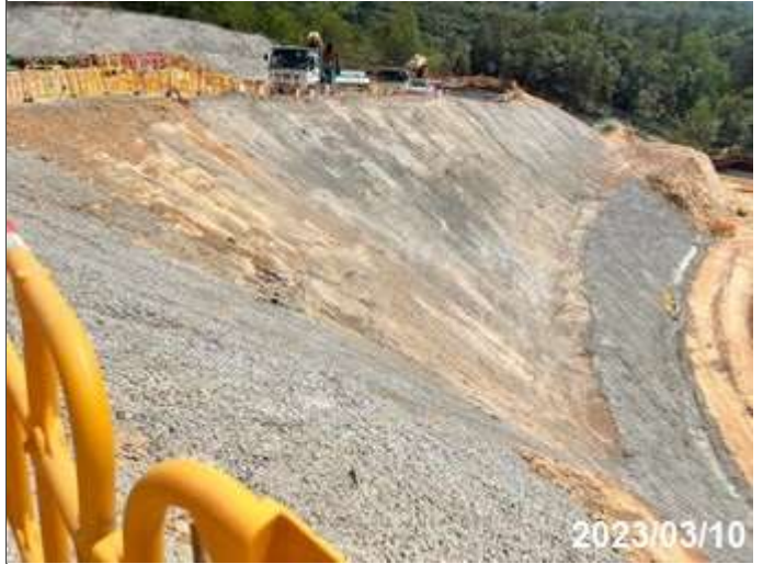
Photo 12 Application of cement slurry at Portion A
