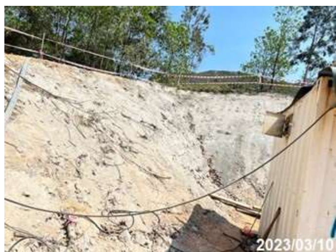
Photo 12 Application of cement slurry at Portion A
