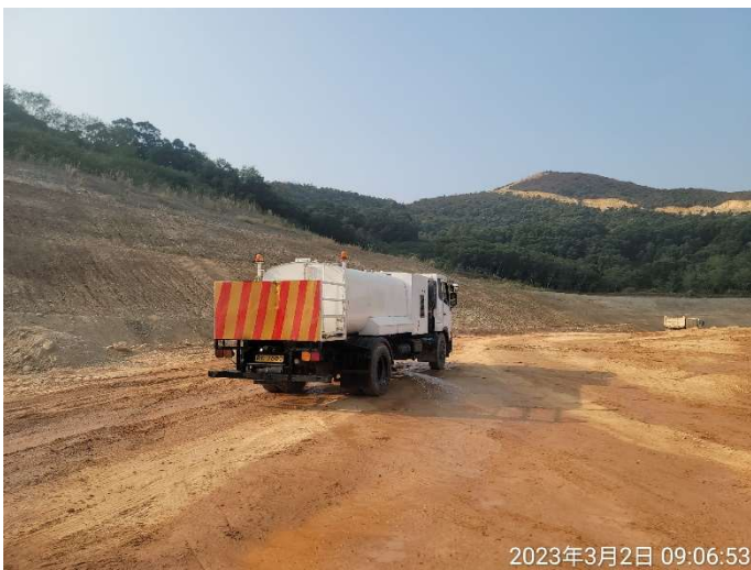
Photo 11 Water spraying by water tanker along the haul road between Portion A and the SBA
