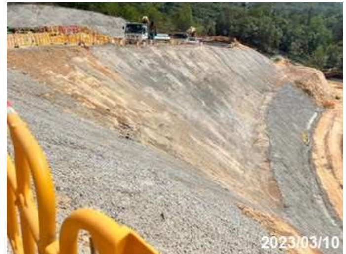
Photo 18 Application of cement slurry at Portion A
