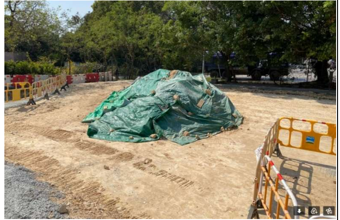
Photo 12 Dusty Materials covered by impervious sheeting at Portion D
