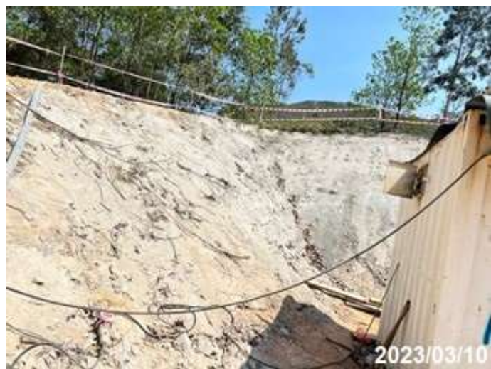
Photo 13 Application of cement slurry at Portion A
