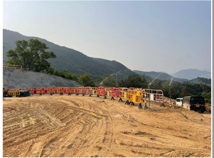
Photo 20 Hydroseeding at bare slope at Portion E3-2 (3 March 2023)
