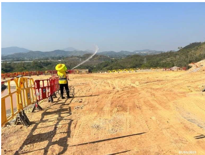
Photo 11 Hydroseeding at bare slope at Portion E3-2 (Implemented start on 26 February 2023)
