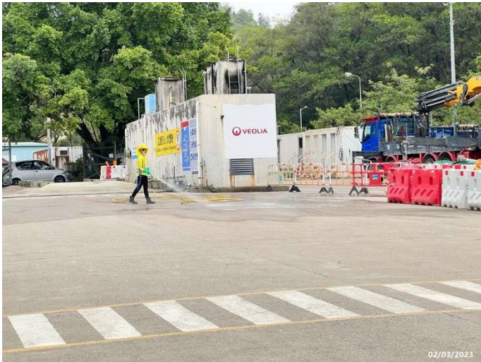
Photo 9 Water spraying by water tanker along the haul road between Portion A and the SBA
