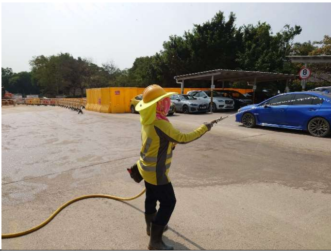
Photo 11 Water spraying by water hose at Portion D
