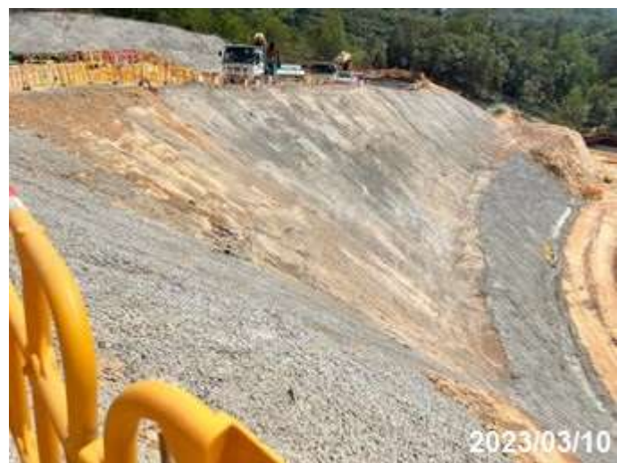
Photo 12 Application of cement slurry at Portion A
