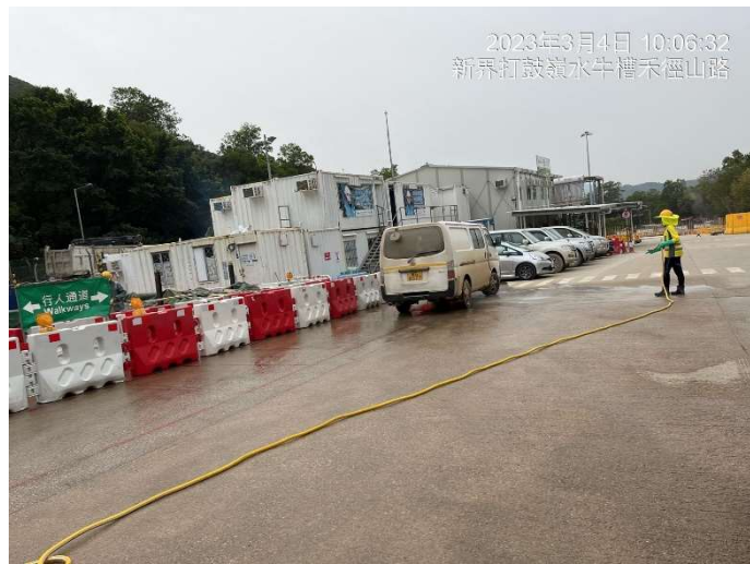
Photo 7 Water spraying by water hose at Portion D
