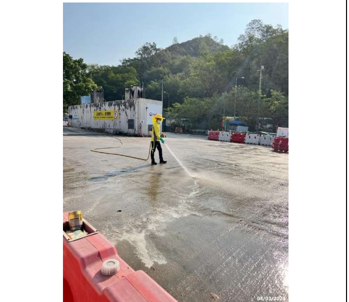
Photo 8 Water spraying by water tanker along the haul road between Portion A and the SBA
