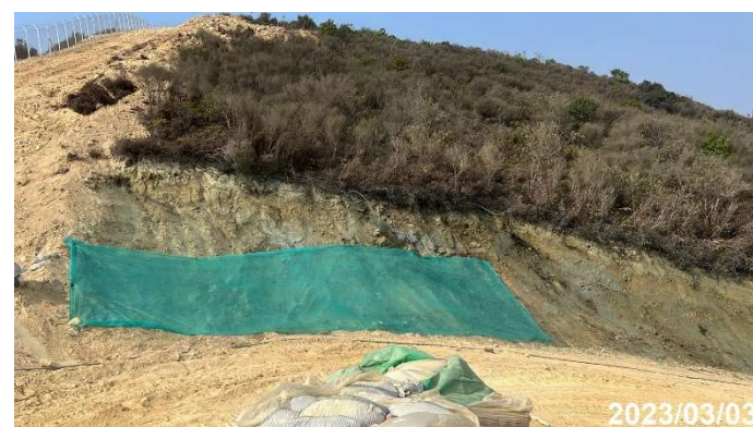
Photo 9 Hydroseeding at bare slope at Portion E3-2
