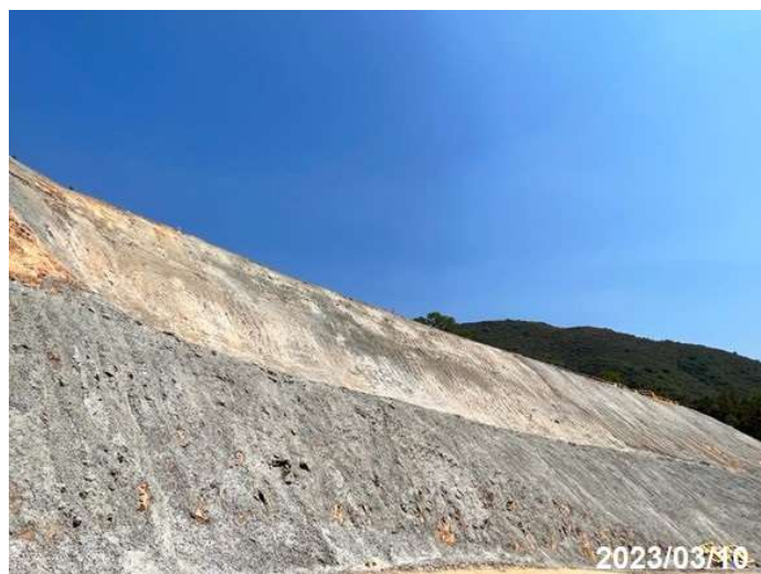
Photo 19 Application of cement slurry at Portion A
