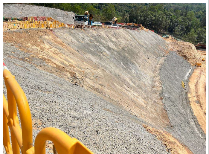
Photo 16 Application of cement slurry at Portion A
