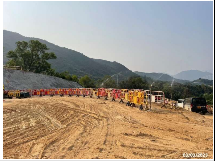
Photo 6 Water spraying by water sprinklers at Portion A
