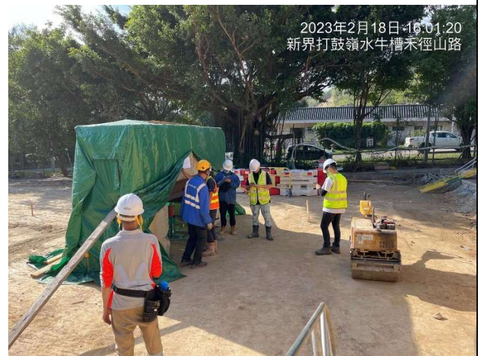
Photo 4 Integrated Building Office (IOB) conducting the plate load test at Portion D
