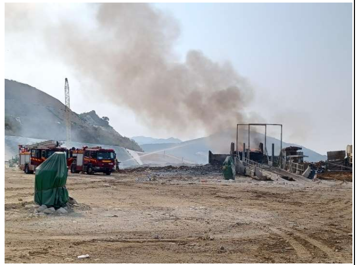
Photo 14 Fire incident near the project site
