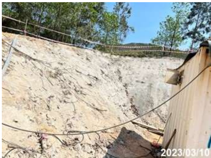
Photo 17 Application of cement slurry at Portion A
