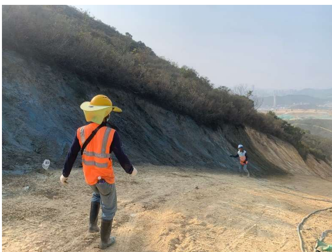
Photo 21 Hydroseeding at bare slope at Portion E3-2 (3 March 2023)
