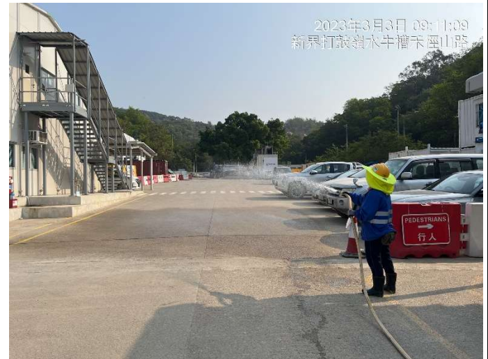
Photo 12 Water spraying by water hose at Portion D
