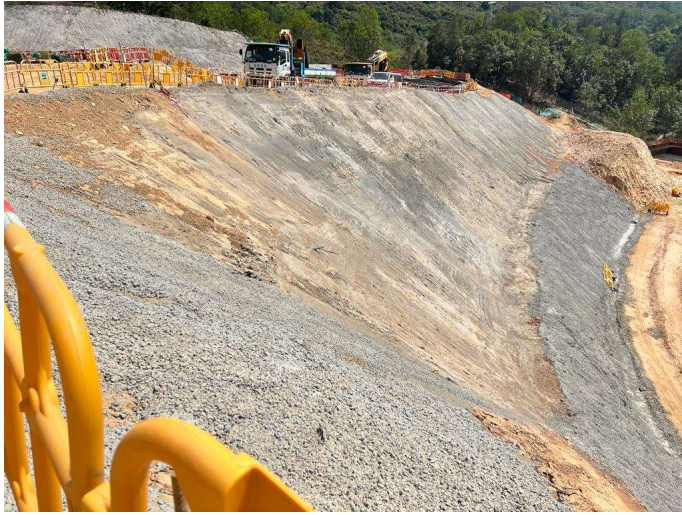
Photo 19 Hydroseeding at bare slope at Portion E3-2 (26 February 2023)
