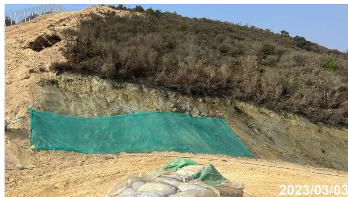
Photo 9 Hydroseeding at bare slope at Portion E3-2
