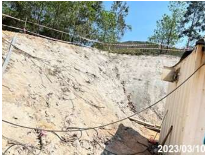
Photo 13 Application of cement slurry at Portion A
