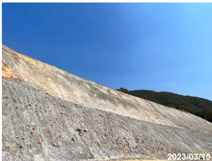
Photo 13 Application of cement slurry at Portion A
