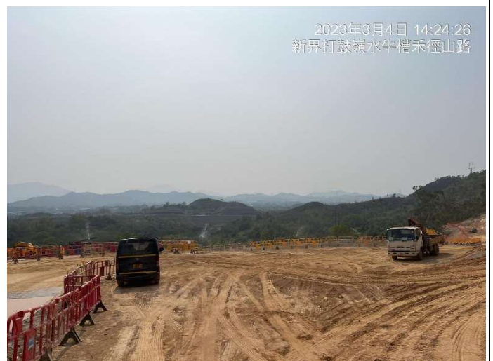
Photo 2 Site formation at Portion A
