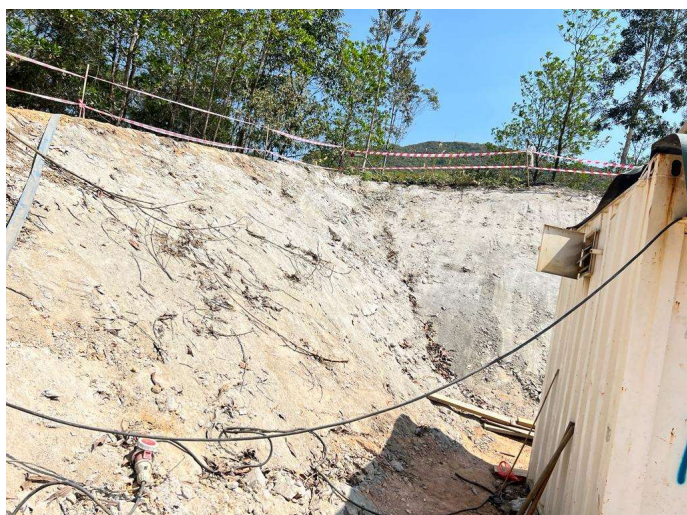
Photo 15 Application of cement slurry at Portion A
