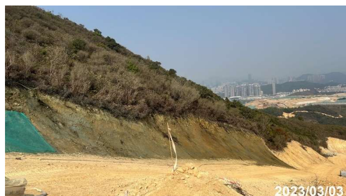
Photo 10 Hydroseeding at bare slope at Portion E3-2
