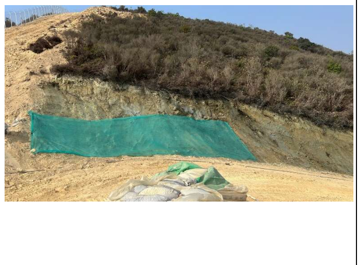
Photo 20 Hydroseeding at bare slope at Portion E3-2 (3 March 2023)
