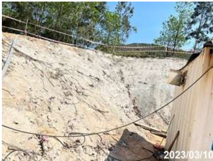
Photo 19 Application of cement slurry at Portion A
