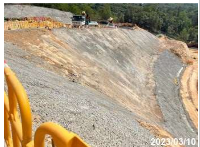
Photo 13 Application of cement slurry at Portion A
