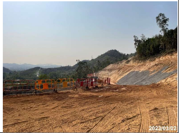
Photo 4 Hydroseeding at Portion E3
