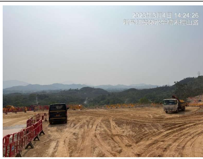
Photo 1 Site Formation at Portion A
