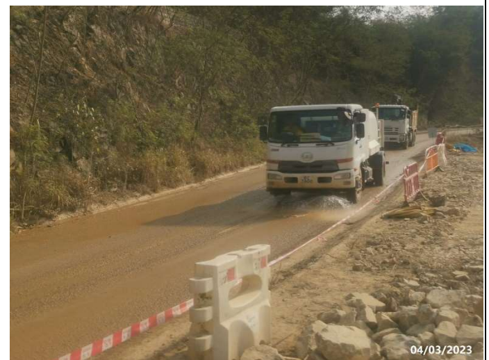
Photo 8 Water spraying by water tanker along the haul road between Portion A and the SBA
