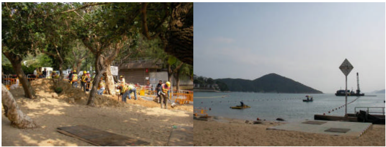
Figure 2.2 General view of the Construction Site (16 March 2009)
