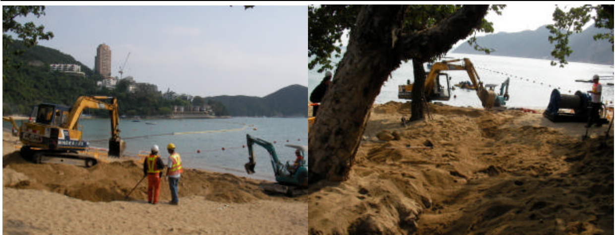
Figure 3.3 Trench Excavation and Backfilling (16 March 2009)
