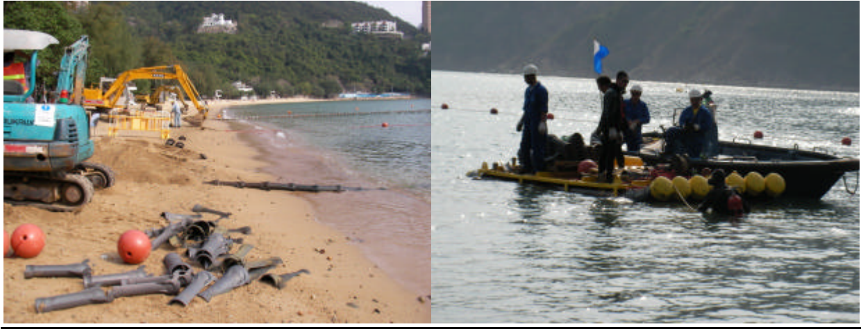
Figure 4.4 Installation of Articulating Pipes (16 March 2009)
