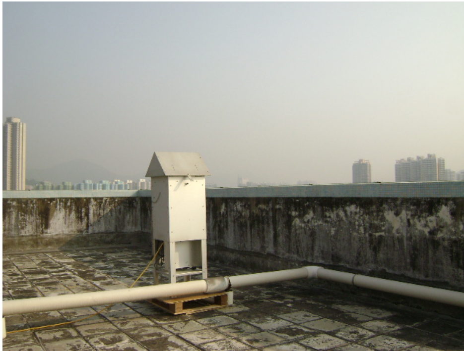
Roof top of Block 15, Yuet Wu Villa
