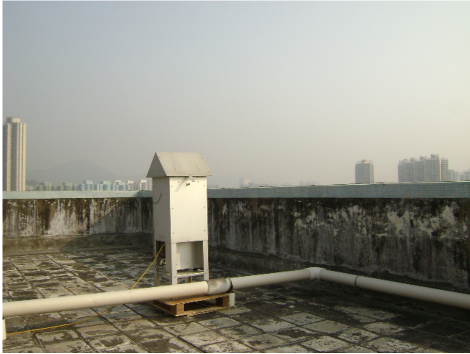
Roof top of Block 15, Yuet Wu Villa
