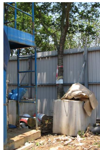
Photo 12 – No proper Tree Protection Zone (T250 as an example in Area A)
