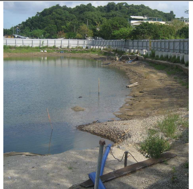
Photo 4. Water intake at fish pond – Area C
