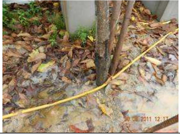
Photo 14 - A sink of water was formed with the grade lowered at the root flares of the relocated trees U34, U35, U36 and U37.
