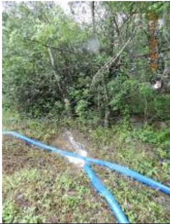
Photo 1 - Water leakage from a drainage pipe was found on the adjacent wasteground next to Area A
