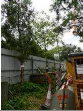
Photo 13 - No proper Tree Protection Zones were established for the highlighted trees in Area A.
