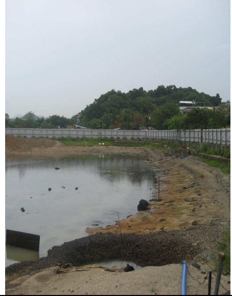
Photo 2. Water intake at fish pond – Area C
