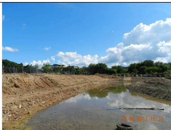
Photo 2 – Landforming and shaping of the southeastern boundary of the ECA were completed as seen from the site inspection on 18th August 2011.
