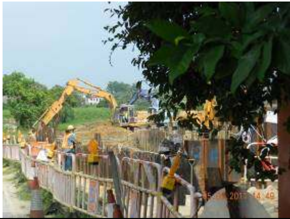
Photo 1 – Temporary hoardings have been erected around the active works area
