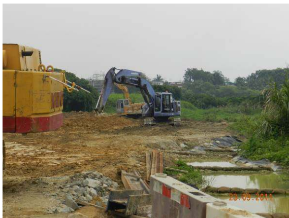
Photo 5 – Clearance of herbaceous vegetation was observed within the active works area.
