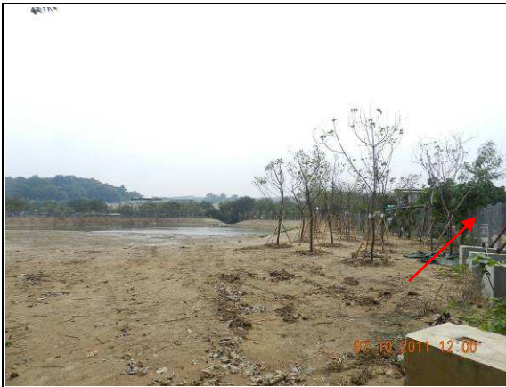
Photo 1 – The chain link fences were established to surround Area C.
