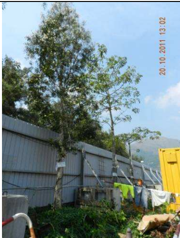
Photo 5 – No proper TPZs were established to protect trees E16 to E20 in Area A
