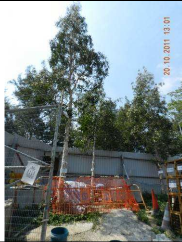
Photo 4 – No proper TPZs were established to protect trees E16 to E20 in Area A
