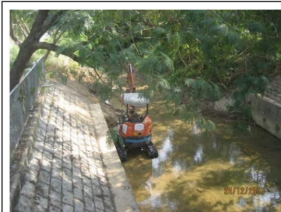
Photo7. Excavation Works from other construction site at upstream
