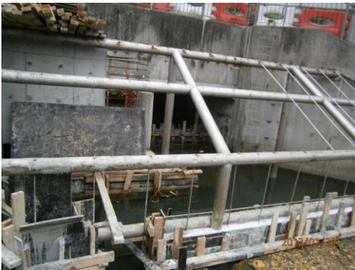
Photo5. One river outlet was closed off for installation of mechanical penstock
